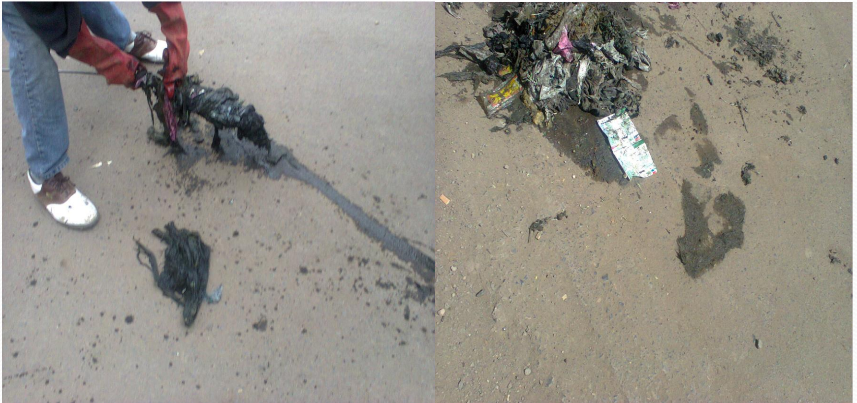
Plate No.1 & 2 showing the materials that are removed from inspection chambers after unblocking of the sewerage system
